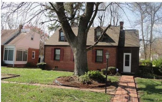
All-brick, solid structure!
